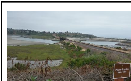
Dredge area: lagoon basin east of the railroad tracks. Photo by Fred Sandquist.
